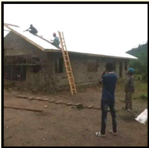
Church Construction Liberia
